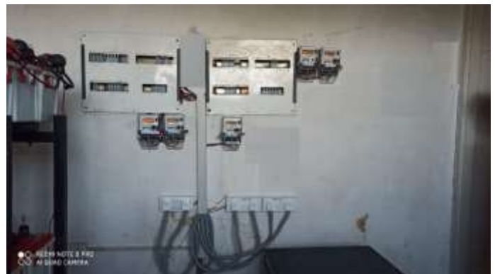
Fig: UPS Loading sharing setup in Admin Ground Floor
